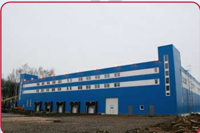
Administrative and warehouse complex S=8000 sq.m. Klimovsk, Moscow region.
